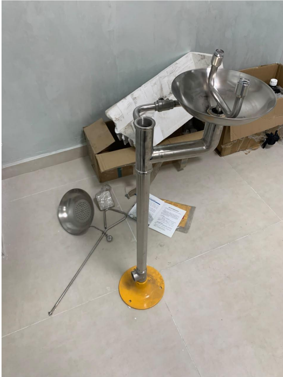
Figure 2.1.6j: Stainless steel floor-mounted Emergency Eyewash and Safety Shower Unit during final assembly and plumbing connection.
